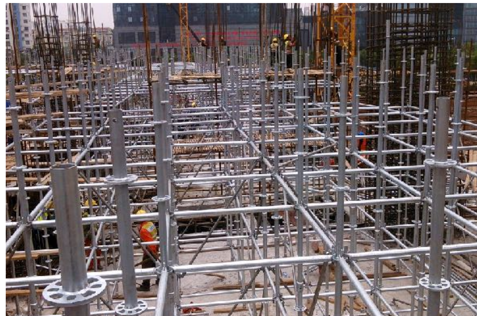
RINGLOCK SHUTTERING SUPPORT IN SHENZHEN
