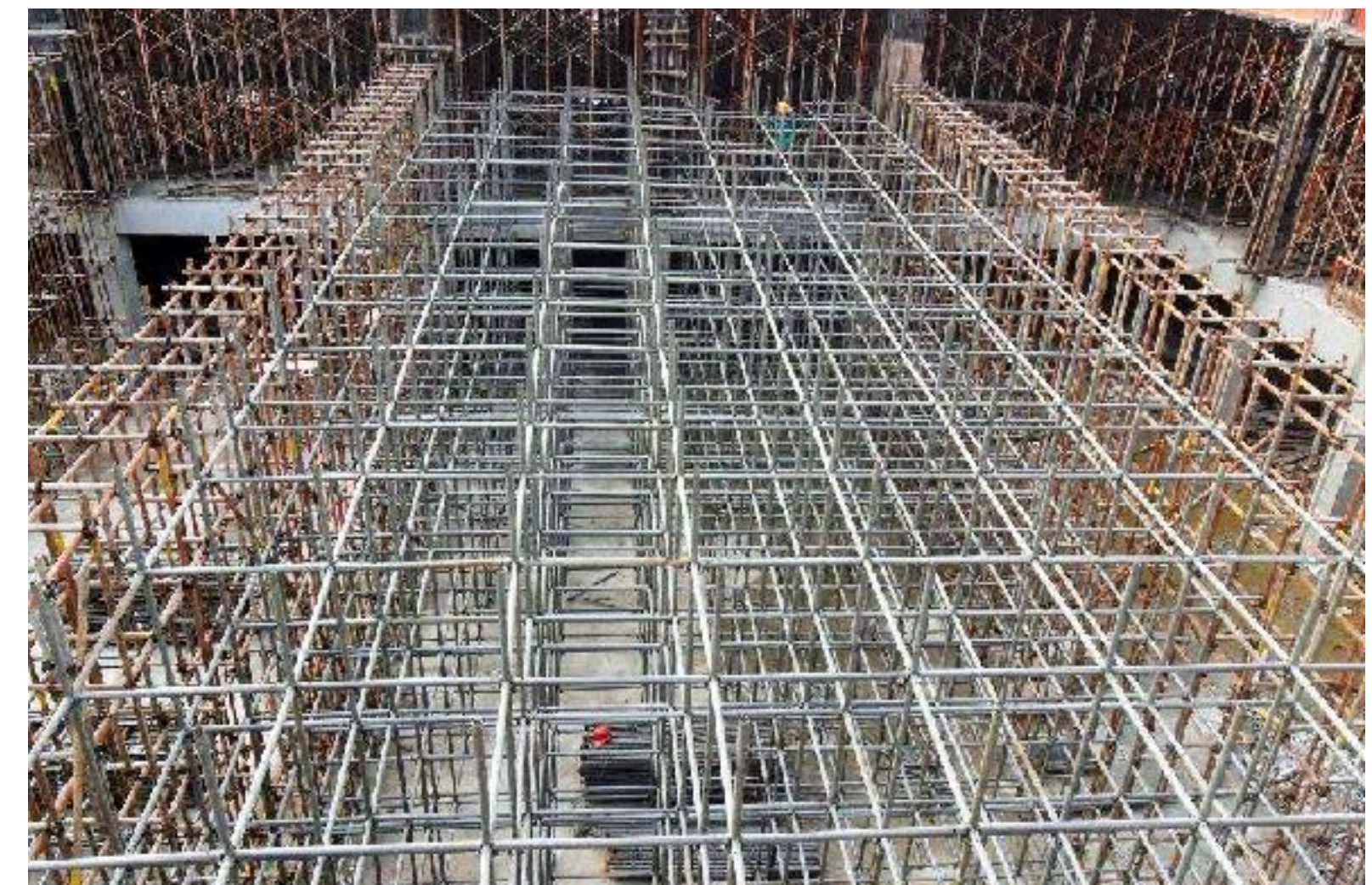
RINGLOCK SHUTTERING SUPPORT IN KENYA
